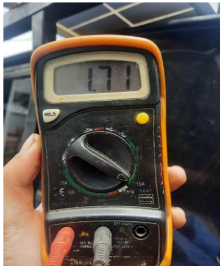
Gambar 9. Pengukuran arus panel surya
