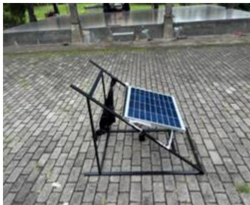
Gambar 6 Lokasi Purwarupa PLTS Ground Mounted
